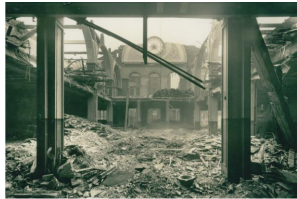
8 The Pantheon demolition 1937
