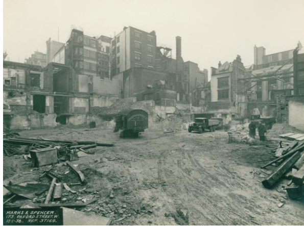
7 M&S Pantheon construction site 1938
