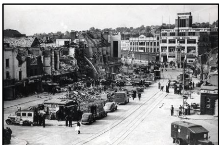
Store damage at Lewisham store, 1944
